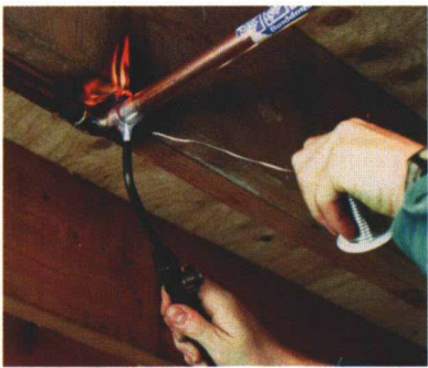
Torch flames often set surrounding wood on fire. Anyone working with a torch should make sure that smoldering embers don't start a blaze after the work is complete.
